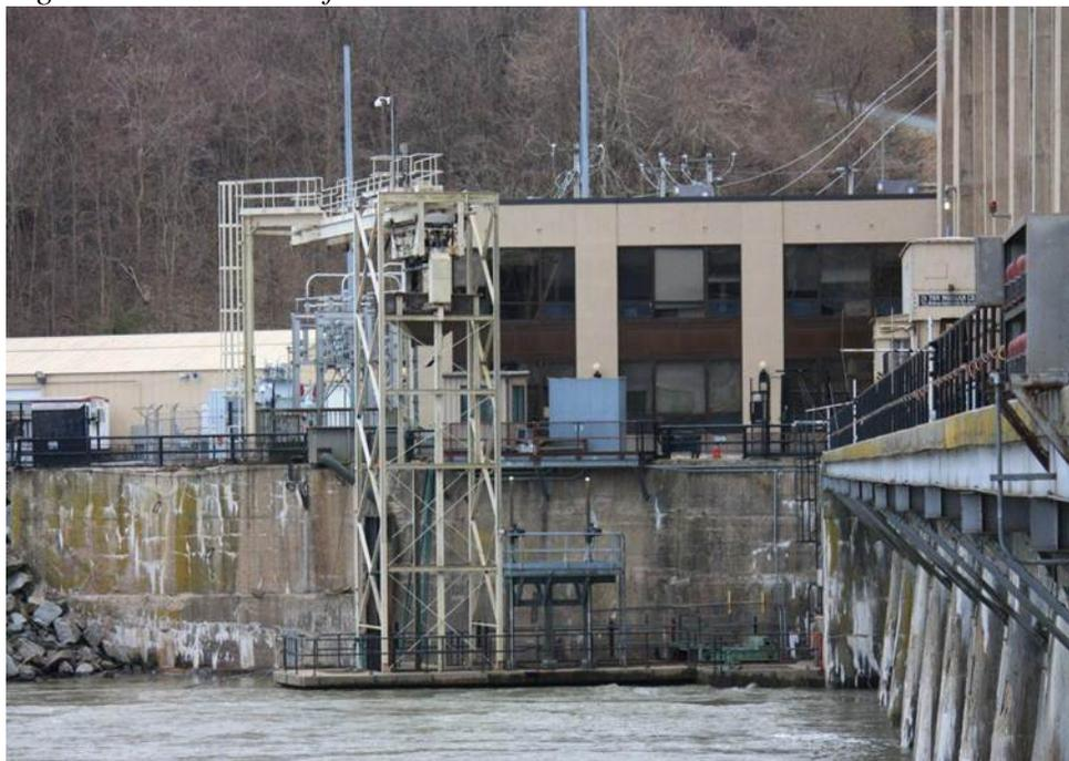
A 1989 Settlement Agreement with the resource agencies resulted in the construction of the East Fish Lift in 1991. The East Fish Lift (Figure 3) is much larger than the West Fish Lift and was
